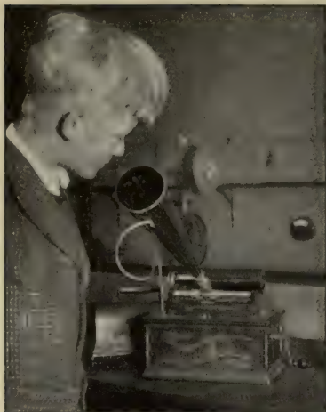
FIG. 98. Making a phonograph record on an old-fashioned phonograph.
